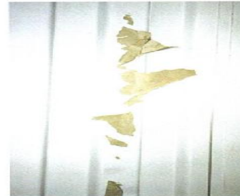
CONDITION PHOTO 6.56/Lining paper remaining on walls that would not be acceptable to a shipper or lessee for shipment of cargo.
