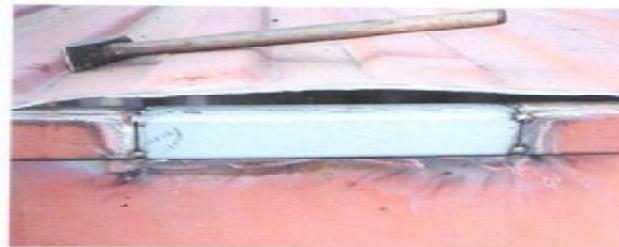
Photo 2.15 / Tube-type top side rail section tack-welded into position
