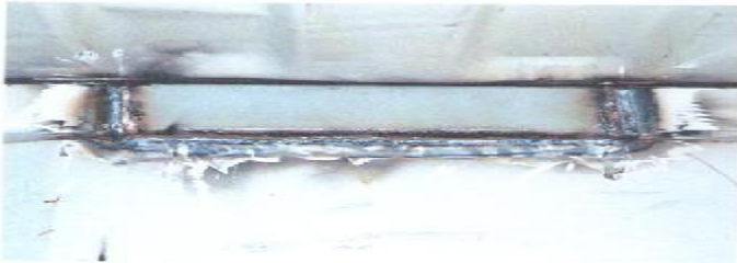
Photo 2.17 / Tube-type top side rail section continuously welded (interior view)
