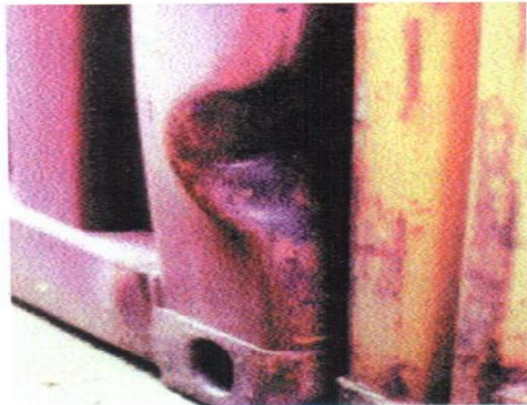
REPAIR REQUIRED Corner post dented more than 25 mm (1 in).
