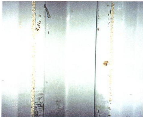
CONDITION PHOTO 6.53/Organic residues stuck to caulking. All organic materials in the container must be removed.
