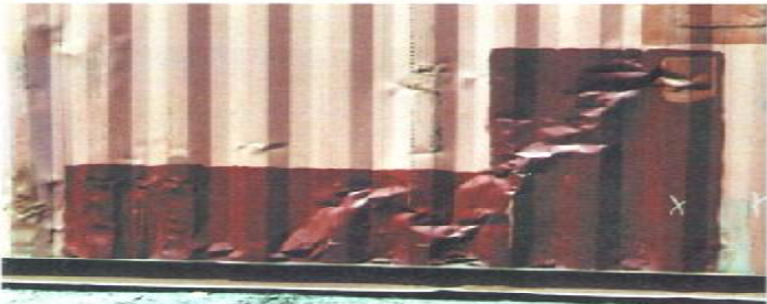
Photo 6.4 / Example of poor panel straightening. The damaged area has been painted, but no attempt has been made to straighten the dents.
