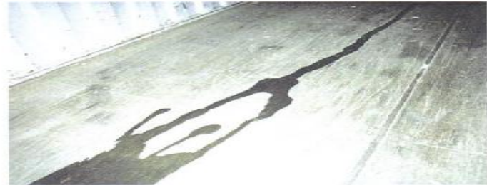
CONDITION PHOTO 6.18/Wet, standing and pooled liquid that would damage cargo.
