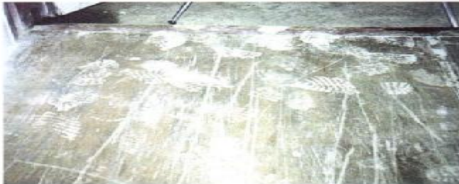
CONDITION PHOTO 6.7/Raised mud foot prints (i.e., footprints having a discernable thickness) in excess of what normally would remain after a sweep out.
