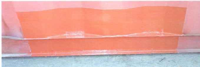
Photo 2.33 / Top coating of bottom rail section completed.
