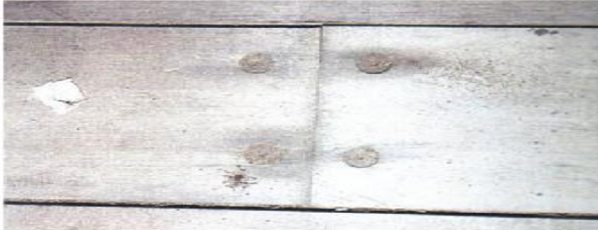
CONDITION PHOTO 6.31/Floor screw corrosion that will not damage dry-van general cargo.
