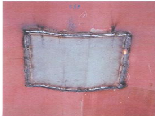
Photo 2.8 / Panel insert continuously welded
