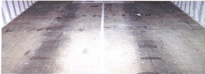
CONDITION PHOTO 6.19 /Forklift tire marks on floor that would not damage dry-van general cargo.
