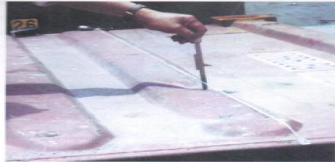
Measuring downward damage on a standing roof corrugation: the inspector measures the distance from reference line to point of maximum downward deflection. Note that the reference line extends along the corrugation across the full width of the roof. See Section 4.6.1.
