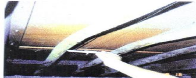
REPAIR REQUIRED Crossmember web deformed more than 50 mm (2 in).
