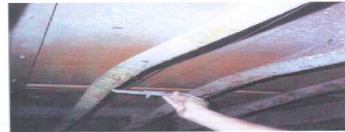
Measuring direct impact to crossmember web: as in the photo on the top of the page, the inspector has extended the reference line along the full width of the crossmember from rail to rail, and is measuring the distance from reference line to maximum point of the web deflection. See Section 4.8.1.
