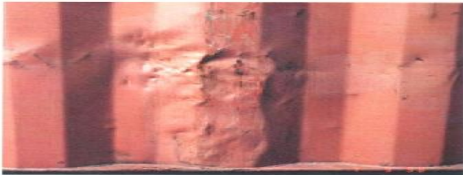
Photo 4.16 Borderline-quality panel straightening. Numerous hammer marks and only a feeble attempt made to restore corrugation profile. The need to rework is dependent on owner's policies.
