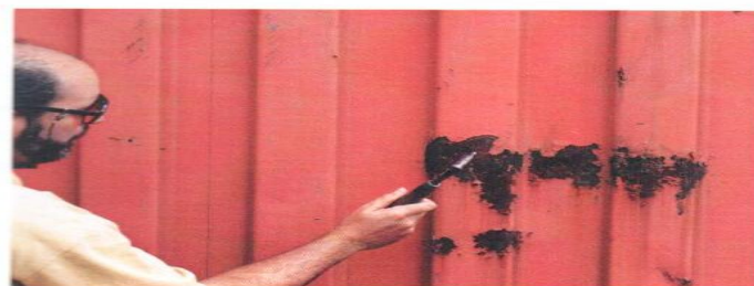
Photo 4.10 Use of the inspector's hammer; if the corroded area shown permanently deforms or becomes holed when struck by a short series of light blows from the hammer, repair is necessary. This is a wear condition. If there is no deformation or holing, no repair is required.
