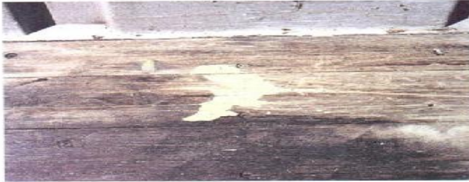
CONDITION PHOTO 6.27/Paint spills that will not transfer to cargo.
