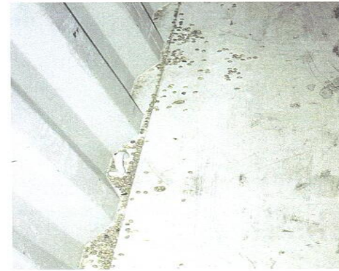
CONDITION PHOTO 6.24/Organic residue on floor. All organic materials inside the container must be removed.
