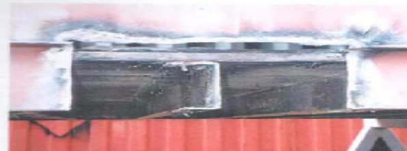
Photo 5.7 / Removal of damaged portion of bottom side rail. Note cutting of welds to side panel beyond the removed area of rail.
