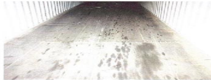
CONDITION PHOTO 6.12/Transferable or non-transferable dried floor stains that will not damage dry-van cargo.
