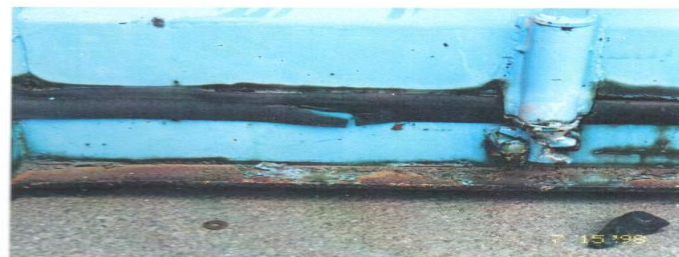
Photo 4.9 Bottom horizontal gasket with cuts. This gasket does not require repair as long as it is still watertight.
