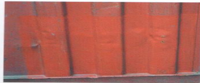
Photo 6.2 / Example of fair panel straightening, with fair corrugation profile and more serious hammer marks
