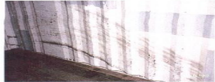
CONDITION PHOTO 6.48 /Non-transferable wall stains that would be acceptable for shipment of dry-van general cargo.
