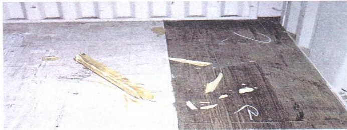
CONDITION PHOTO 6.25/ Debris and dunnage that would damage dry-van general cargo and impede the safe loading and operation of the container.
