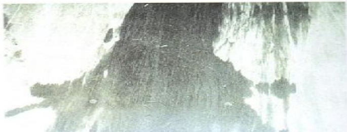
CONDITION PHOTO 6.15 /Transferable, damp, liquid stain that would damage dry-van general cargo.
