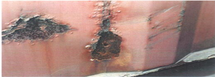
Photo 4.11 Corroded area holed by the inspector's hammer test. This is a wear condition which must be repaired.
