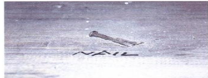
CONDITION PHOTO 6.34/Nails protruding above floor surface which will damage dry-van general cargo and impede the safe loading and operation of the container.
