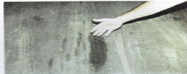
CONDITION PHOTO 6.8/Dry dust covering dried floor stains as would normally remain after a sweep out.
