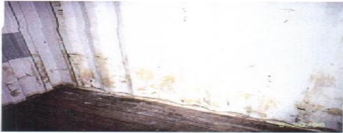
CONDITION PHOTO 6.47 /Non-transferable wall stains that would be acceptable for shipment of dry-van general cargo.
