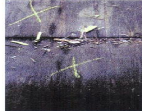
REPAIR REQUIRED Heights of adjacent plywood panels differ by more than 5 mm (3/16 in).
