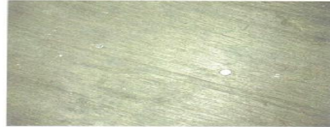
CONDITION PHOTO 6.32/Nail heads that are flush to surface and will not damage dry-van general cargo and will not impede the safe loading and operation of the container.
