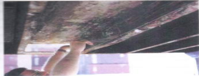
Measuring direct impact to crossmember web: the inspector measures the distance from reference line to point of maximum deflection in the web. Note that the reference line extends across the full width of the crossmember along the formed edge between web and flange. See Section 4.8.1.
