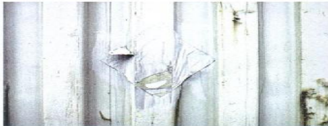
CONDITION PHOTO 6.73/Painted-over labels that would not be acceptable for shipment of dry-van cargo.
