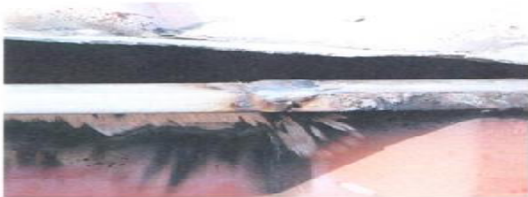
Photo 5.5 / Welding of flat-bar top side rail section to original rail (third pass)
