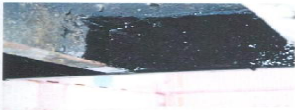
Photo 5.9 / Undercoating bottom rail section (primer was applied beforehand)
