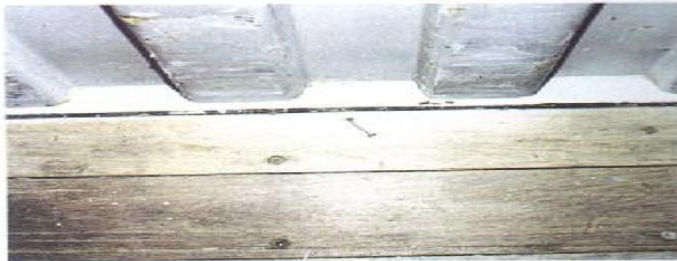
CONDITION PHOTO 6.33/Nails protruding above floor which could damage dry-van general cargo and could impede the safe loading and operation of the container.
