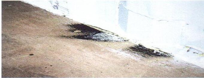
CONDITION PHOTO 6.29/Transferable burn marks on floor that will not damage dry-van general cargo.
