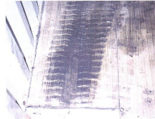
CONDITION PHOTO 6.20 /Forklift tire marks on floor that would not damage dry-van general cargo.
