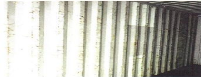
CONDITION PHOTO 6.36/Accumulated scratches due to normal use of container.
