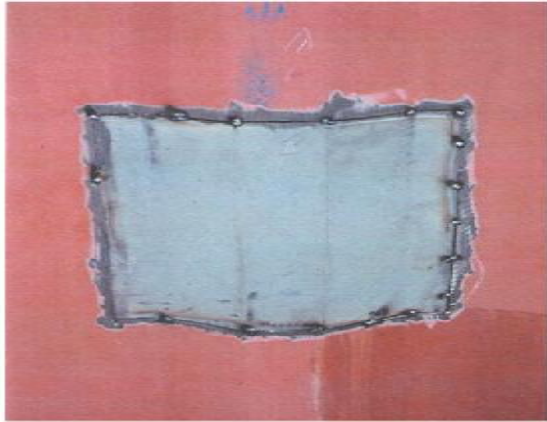
Photo 2.7 / Panel insert tack welded in position
