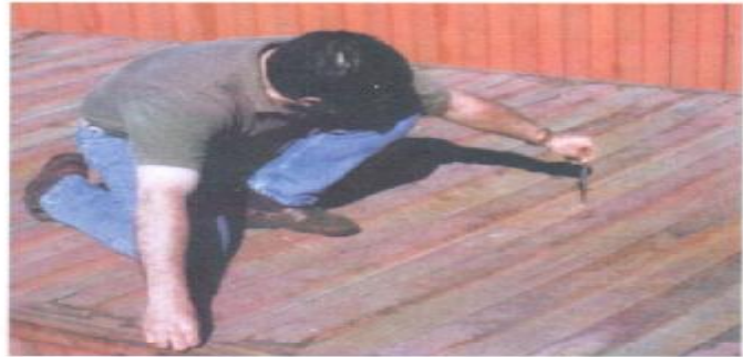
Measuring downward damage on the flat panel area between corrugations: the inspector measures the distance from reference line to point of maximum downward deflection. Note that the reference line has been placed on the flat panel area between corrugations, and extends across the full width of the roof. See Section 4.6.2.
