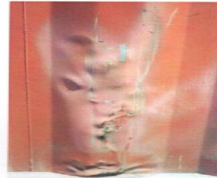
Photo 4.17 Poor-quality panel straightening. Only a feeble attempt made to restore corrugation profile, using a large-headed hammer without a corrugation dolly. There is significant stretching of metal. No attempt at surface preparation has been made. Rework subject to owner's policies.
