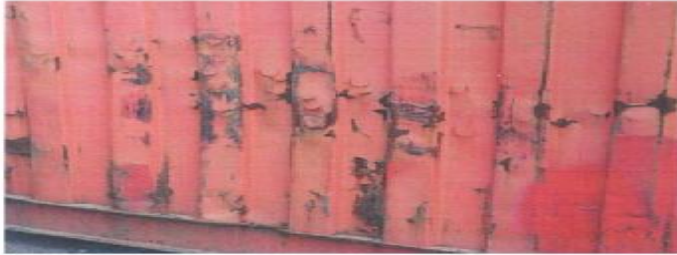
Photo 4.19 Poor-quality panel straightening. Numerous hammer marks and no surface preparation or painting. Rework required (subject to owner's policies).
