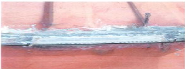
Photo 5.6 / Completed welding of flat-bar top side rail section. A portion of the welds between the section and the original rail has been ground down to permit proper reattachment of the roof sheet.
