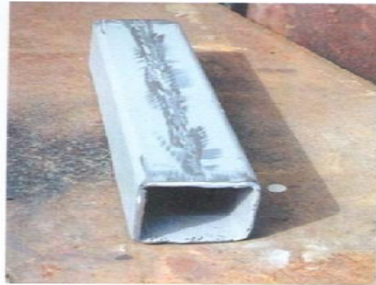
Photo 2.14 / Tube-type top side rail section cut to size, cleaned and beveled
