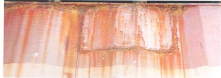
Photo 4.13 Surface corrosion due to improper surface preparation and painting of top side rail and panel patch (exterior). The degree of corrosion does not require repair by itself, although the condition still may be repair-worthy depending on the owner's policy on correcting improper repairs of this type.
