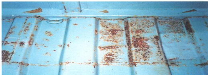
Photo 4.12 Surface corrosion due to improper surface preparation and painting of a panel patch (interior view). The degree of corrosion does not require repair by itself, although the condition still may be repair-worthy depending on the owner's policy on correcting improper repairs of this type.
