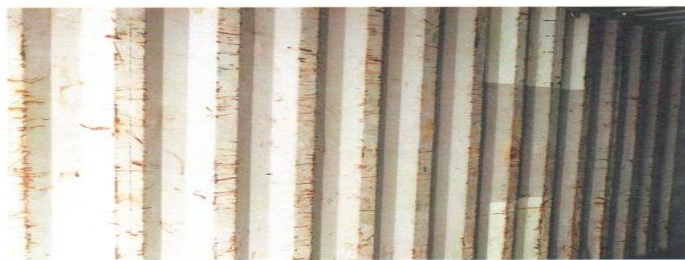
Photo 4.8 Normal-use scratches on standing corrugations. Note the relative absence of scratches on recessed corrugations. This is a wear condition.
