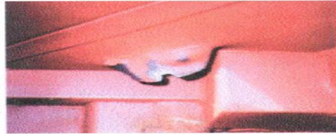
REPAIR REQUIRED Corner protection plate holed.
