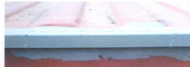
Photo 2.19 / Priming of tube-type top side rail section and adjacent surfaces on the exterior. See note above for Photo 2.18.
