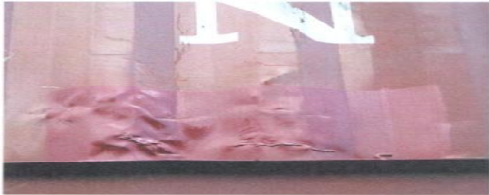
Photo 6.3 / Example of poor panel straightening, with numerous deep hammer marks and poor corrugation profile
