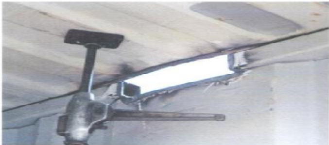
Photo 2.13 / Jacking up of roof sheet to provide clearance for removal of damaged material and rewelding of top side rail section
