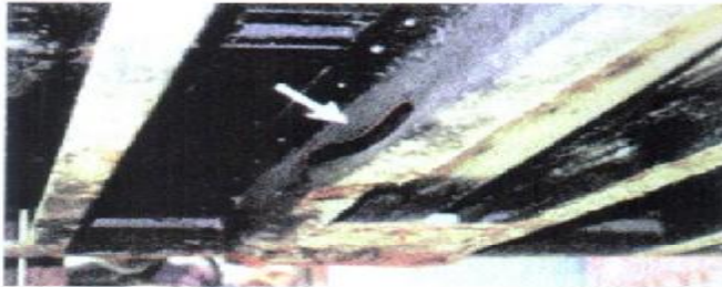
REPAIR REQUIRED Forklift pocket side holed.
