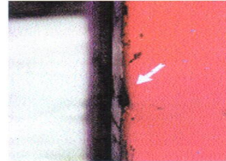
REPAIR REQUIRED Corner post holed.
