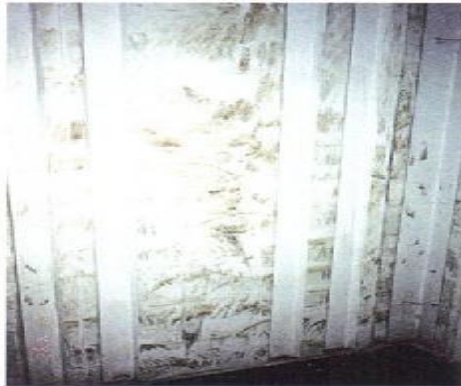
CONDITION PHOTO 6.49/Non-transferable wall stains that would be acceptable for shipment of dry-van general cargo.
