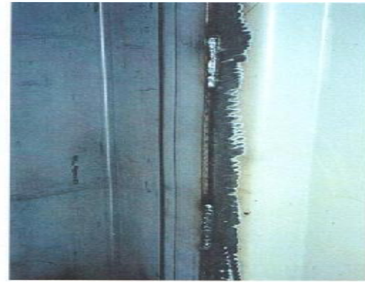
Photo 2.27 / Skip welding of interior of corner post/panel lap joint
