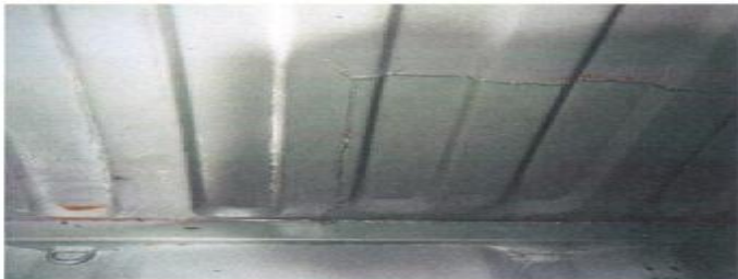
Photo 4.20 Insert to a roof panel with a different corrugation profile at the end. No rework required.
