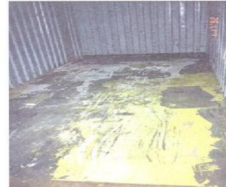
CONDITION PHOTO 6.28/Major paint spillage that would not be acceptable to a shipper or lessee.
