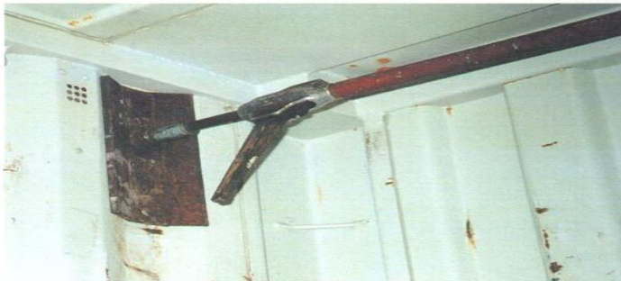
Photo 2.4 / Using a jack with a backing plate to straighten a side panel
