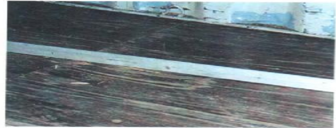
Photo 4.5 Wavy floor is a sign of delamination. Check for accompanying conditions ( e.g. sagging crossmembers under the wavy area) to determine whether this is a damage or wear condition.
