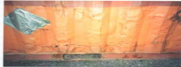
Photo 4.18 Poor-quality panel straightening. No attempt made to restore corrugation profile. Poor-quality painting and paint mismatch. Rework required (subject to owner's policies).
