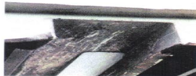
REPAIR REQUIRED Forklift pocket strap missing.
