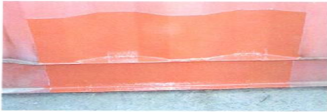
Photo 2.33 / Top coating of bottom rail section completed.
