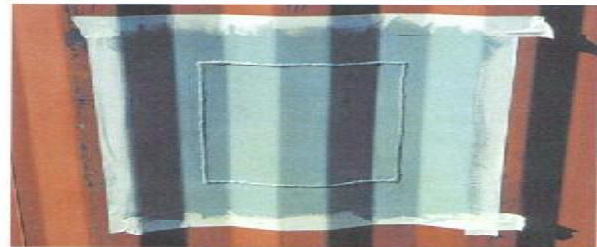
Photo 2.10 / Masking and priming of panel insert repair
