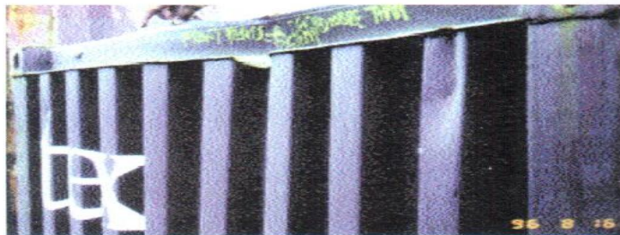
REPAIR REQUIRED Front header deformed more than 25 mm (1 in).
