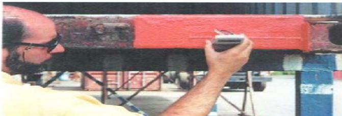
Photo 2.34 / Use of an electronic dry-film paint thickness gauge
