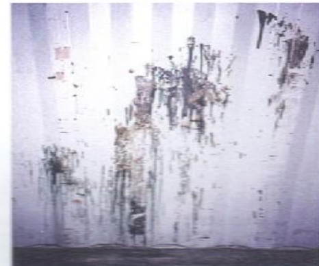
CONDITION PHOTO 6.50/Non-transferable wall stains that would not be acceptable to a shipper or lessee for shipment of dry-van general cargo.
