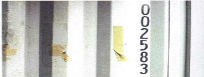
CONDITION PHOTO 6.55/Tape remaining on walls that would not be acceptable to a shipper or lessee for shipment of cargo.
