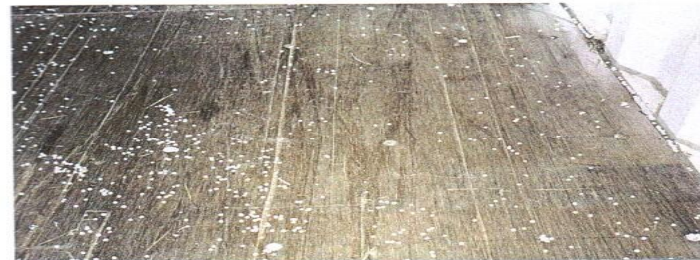
CONDITION PHOTO 6.22 /Polyethylene beads remaining on floor surface and stuck to caulking that would impede the safe loading and operation of a container.
