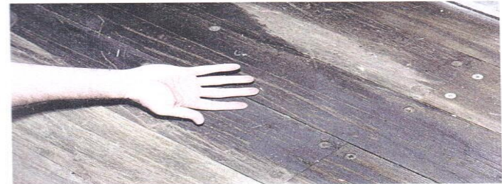
CONDITION PHOTO 6.10/Transferable damp floor stain that would not damage dry-van general cargo.
