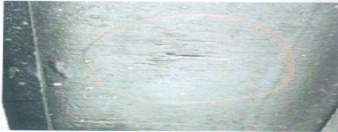
Photo 4.3 Finger crack (in circled area) on underside of floor, directly below the impact shown in Photo 4.2. Since this is accompanied by a sign of impact, this is considered damage .
