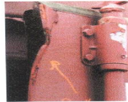
NEED TO REPAIR UNDETERMINED Door panel dented less than 35 mm (1-3/8 in), which does not require repair. However, if door is not both water-tight and light-tight, repair would be required.
