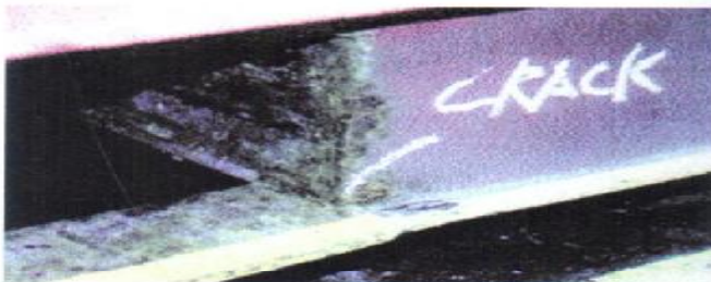
REPAIR REQUIRED Forklift pocket strap weld cracked.
