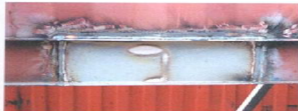
Photo 5.8 / Welding of bottom rail section to original rail, panel and crossmember
