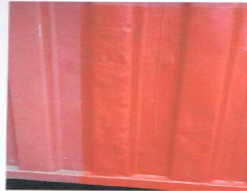
Photo 6.1 / Example of good panel straightening, with well-formed corrugation profile (although with a few hammer marks)
