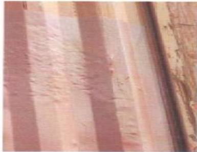
Photo 4.15 Acceptable panel straightening. Despite many hammer marks, the corrugation profile was reasonably restored; rework is not required.
