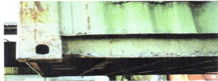
NEED TO REPAIR UNDETERMINED Since dent to bottom side rail is within 250 mm (10 in) of corner fitting, the weld to the fitting must be carefully examined and repaired if there is any evidence of break, cut, tear, crack or other damage.
