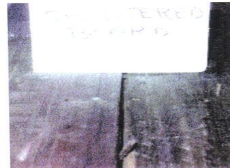
REPAIR REQUIRED Splintered.
