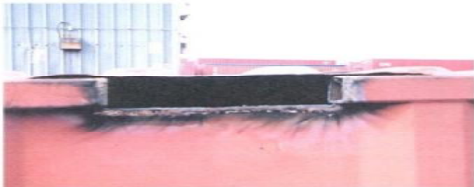
Photo 2.12 / Damaged top side rail area removed before installing a new section. Note that the roof panel has been detached beyond the edges of the removed area, and the edges of rail have been beveled.
