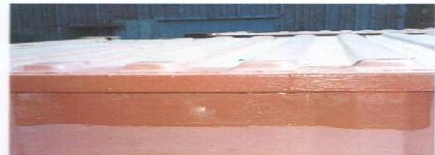
Photo 2.20 / Top-coating of tube-type top side rail section and adjacent surfaces on the exterior. See note above for Photo 2.18.
