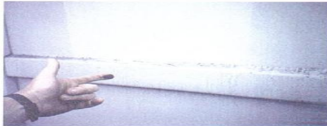
CONDITION PHOTO 6.35/Dust and dirt on walls that will damage dry-van general cargo.
